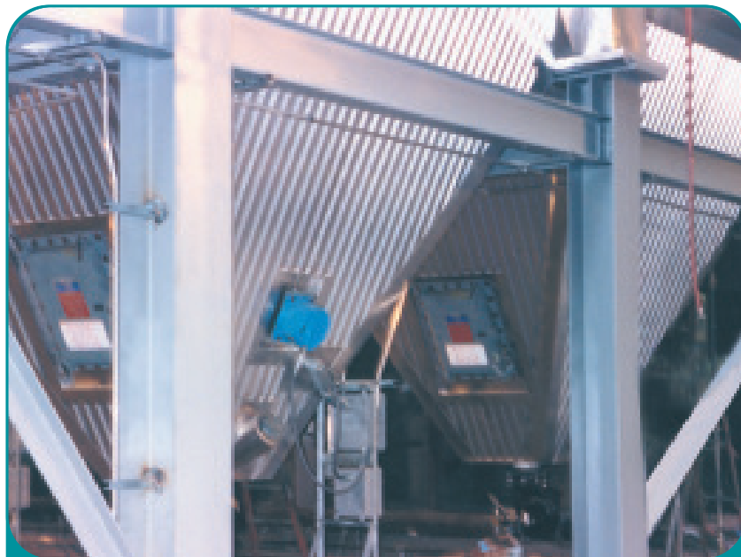
This Syntron® model V-85 Electromagnetic Vibrator is maintaining flow of dust particulates from the collecting hopper of an electrostatic precipitator.
