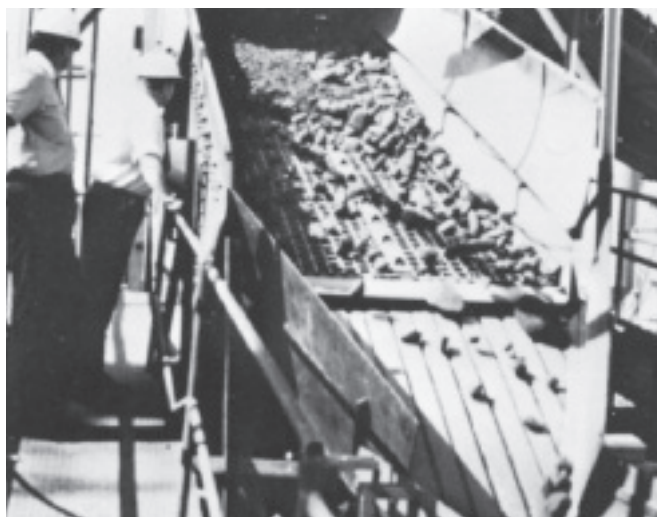
Link-Belt® Model CH two-deck vibrating , 6" wide x 20' long handling rock at 200 TPH.
